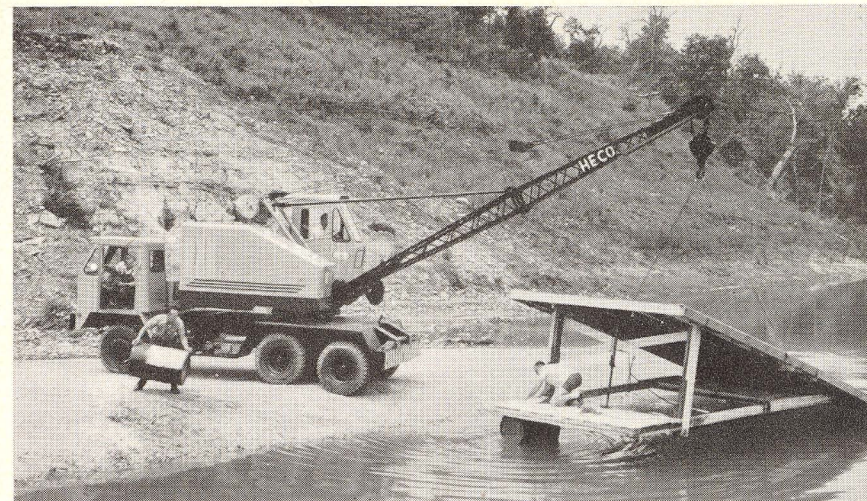
Mechanical muscles, a Heco mobile crane, lifts Texoma club's new ramp into the water.
